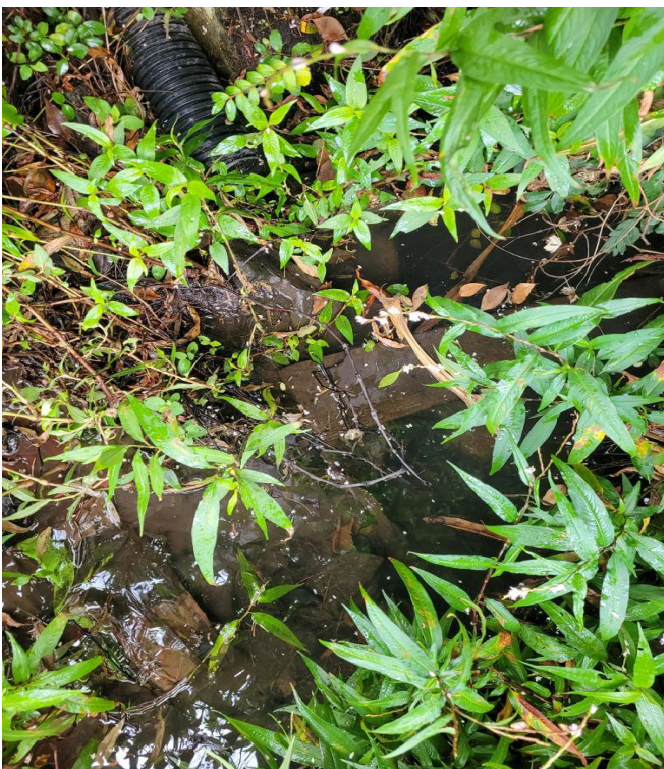
Figure 9: Piped discharge at the artificial reach taken during May 2022 site visit.
