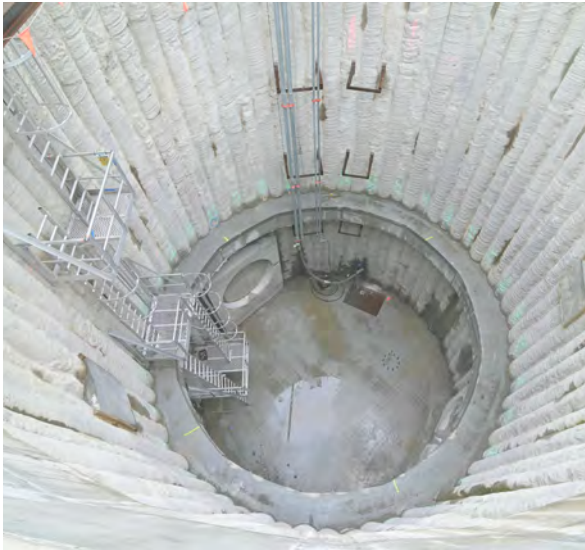
Miranda Reserve shaft
