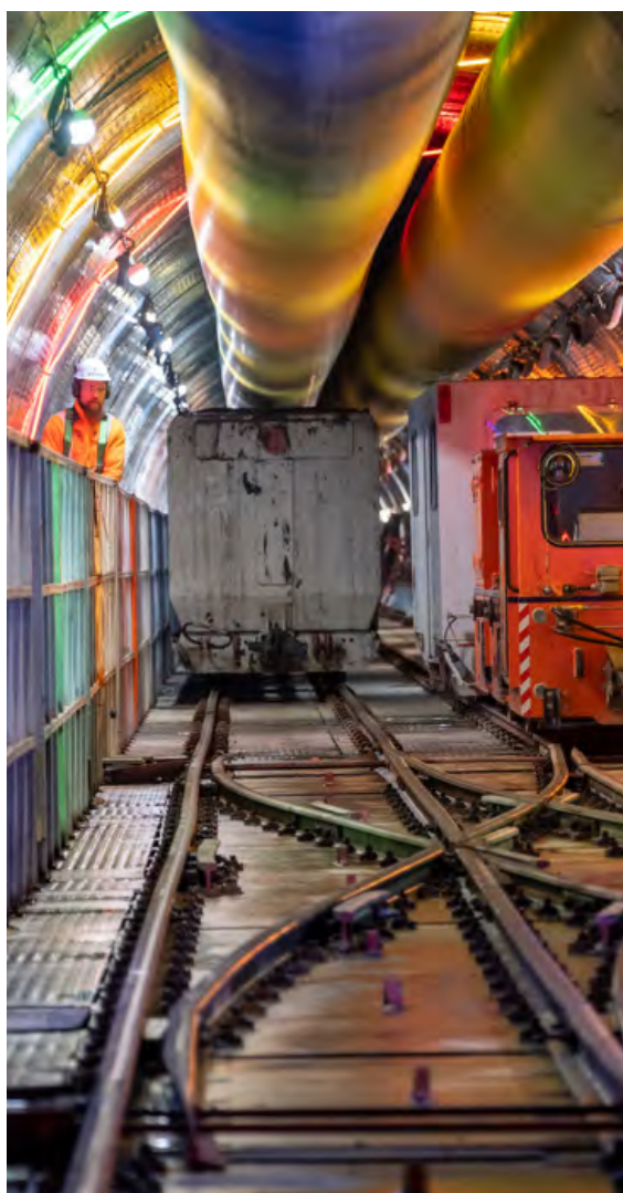
Colour coding the tunnel for safety
