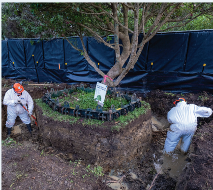
Where we can, we relocate trees from our construction sites, rather than just cut them down
