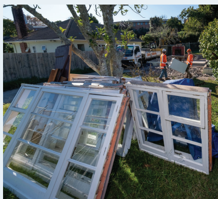
Rather than demolish we deconstruct and recycle
