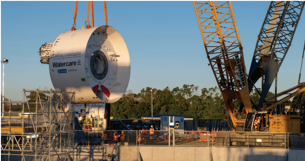
Hiwa-i-te-Rangi about to be lowered underground
