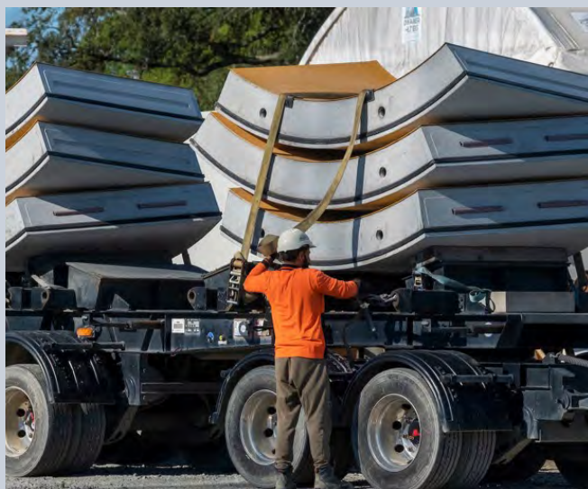
Six segments for just one ring makes a big load
