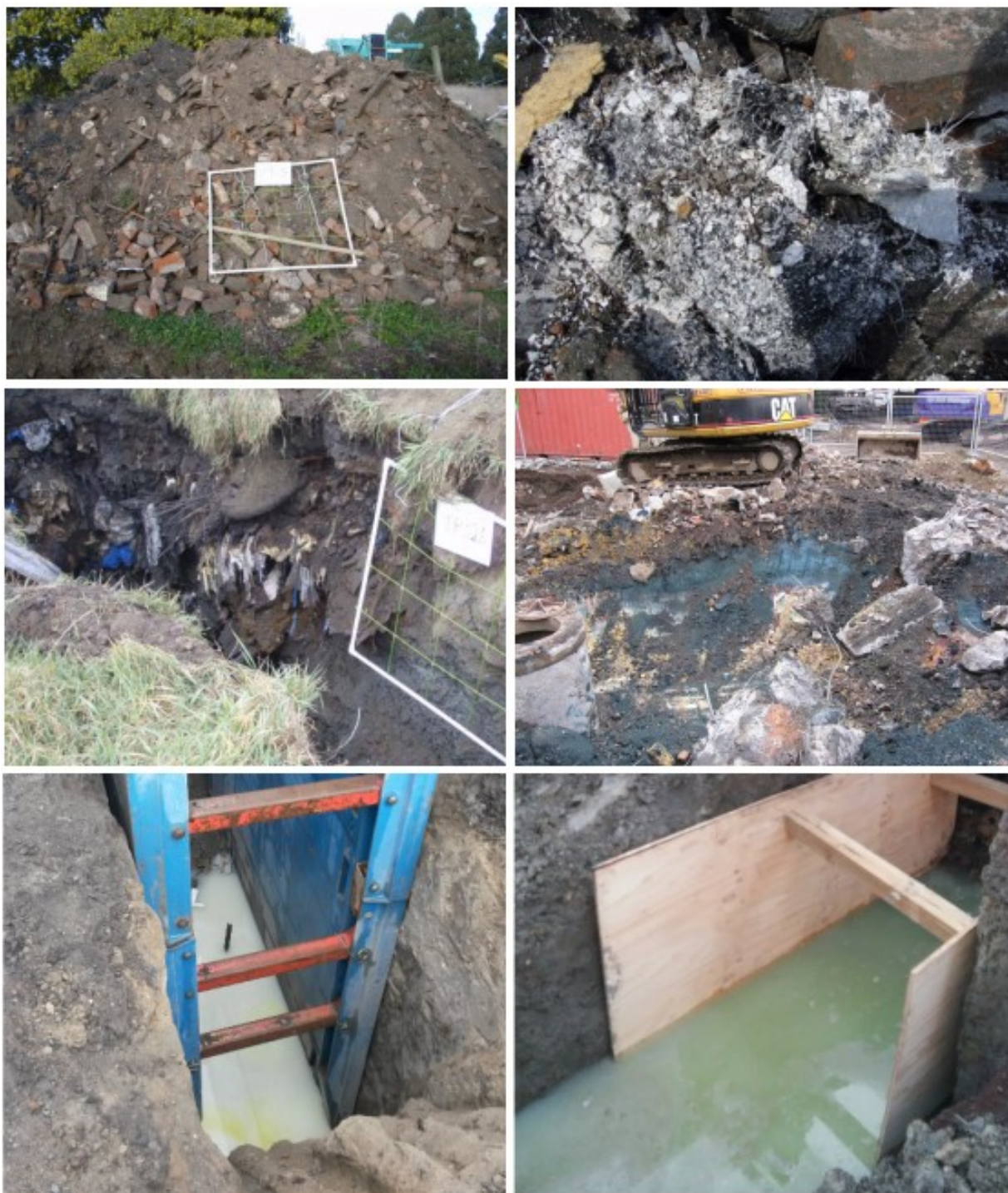
Figure 3: Contamination photos, clockwise from top left: excavated construction rubble; excavated potential ACM; 'blue billy' cyanide staining beneath concrete; green stained groundwater; white stained groundwater; municipal waste filling.
