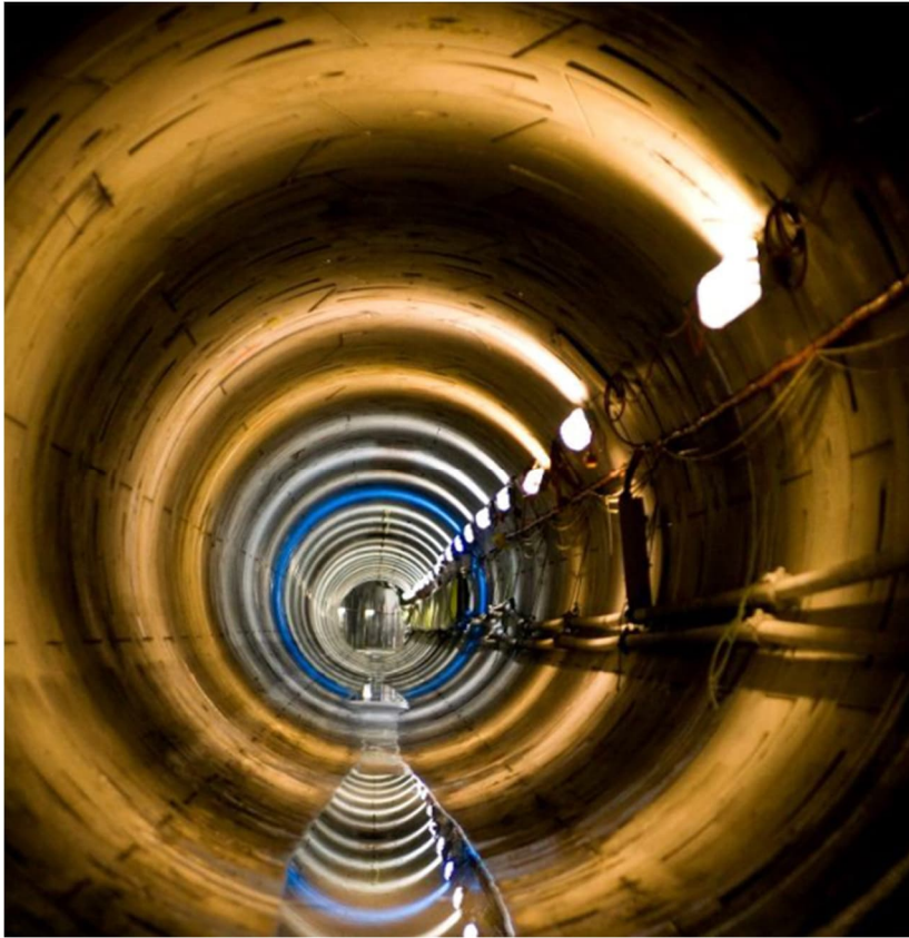
Figure 4.3: Precast Concrete Segmentally Lined Tunnel
