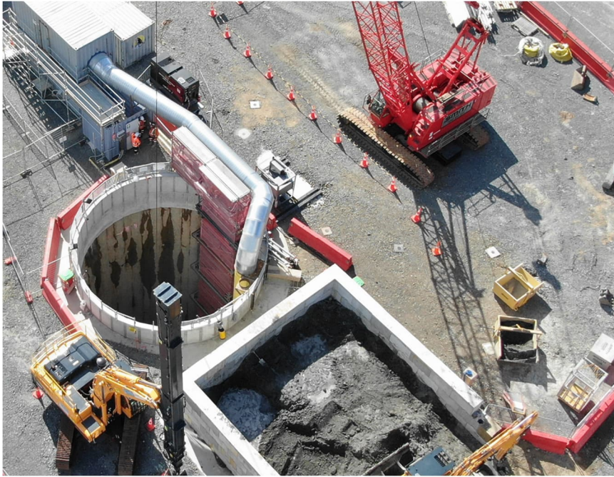
Figure 4.7: Shaft at May Road supported by Secant Piles in overburden Soil and Shotcrete and Mesh in ECBF Rock
