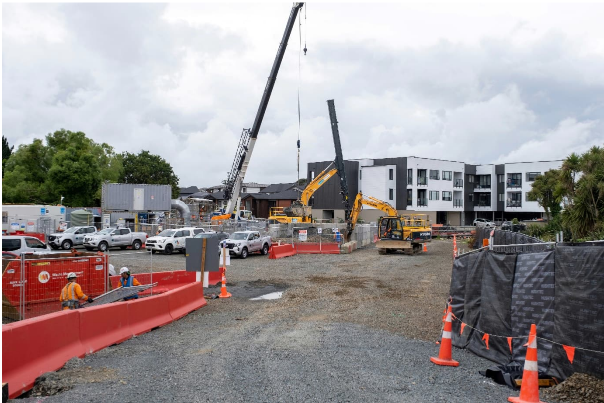
Figure 4.6: Haverstock Shaft Site construction yard
