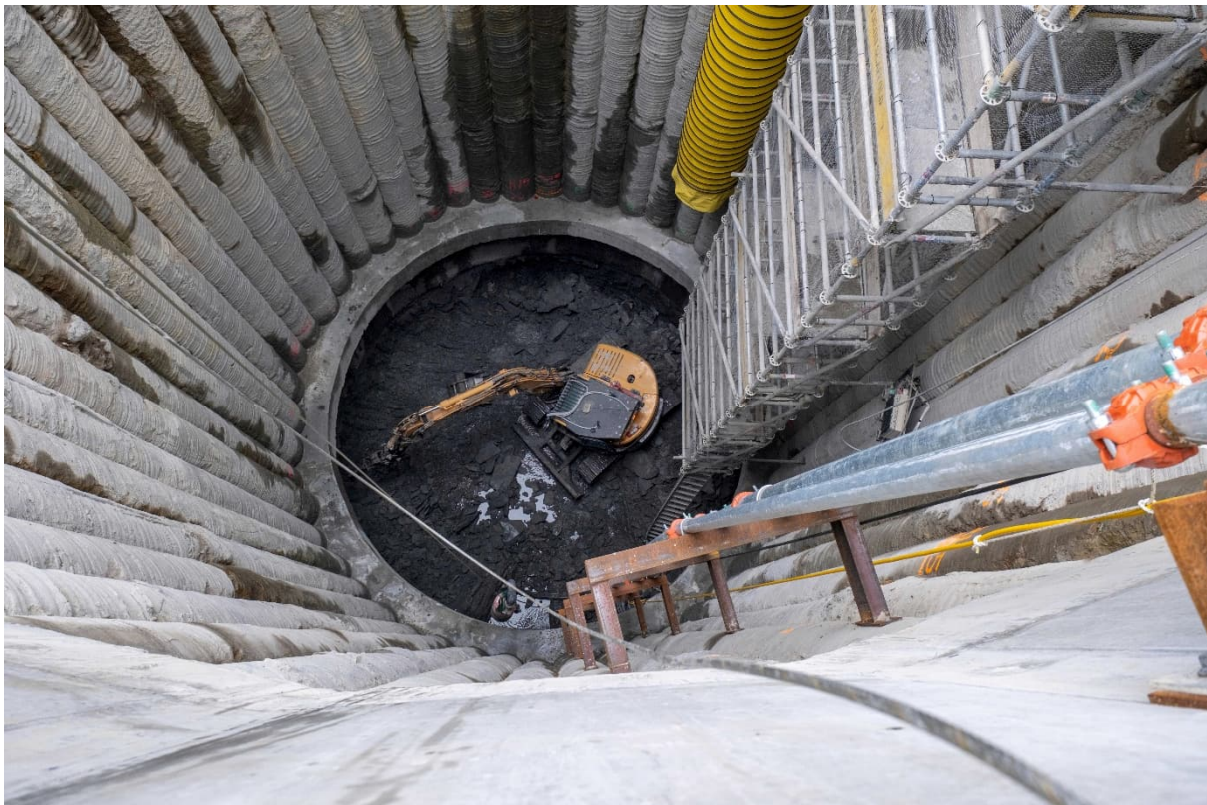
Figure 4.8: Haverstock shaft construction – secant piles
