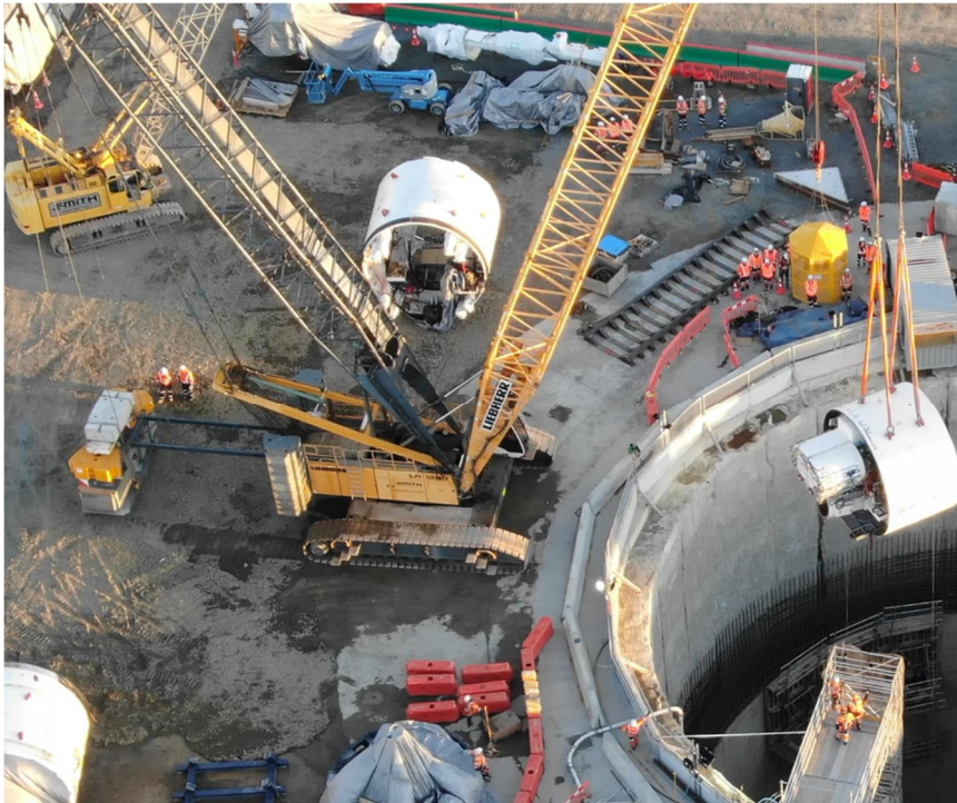
Figure 4.9: TBM installation at Māngere shaft – June 2021
