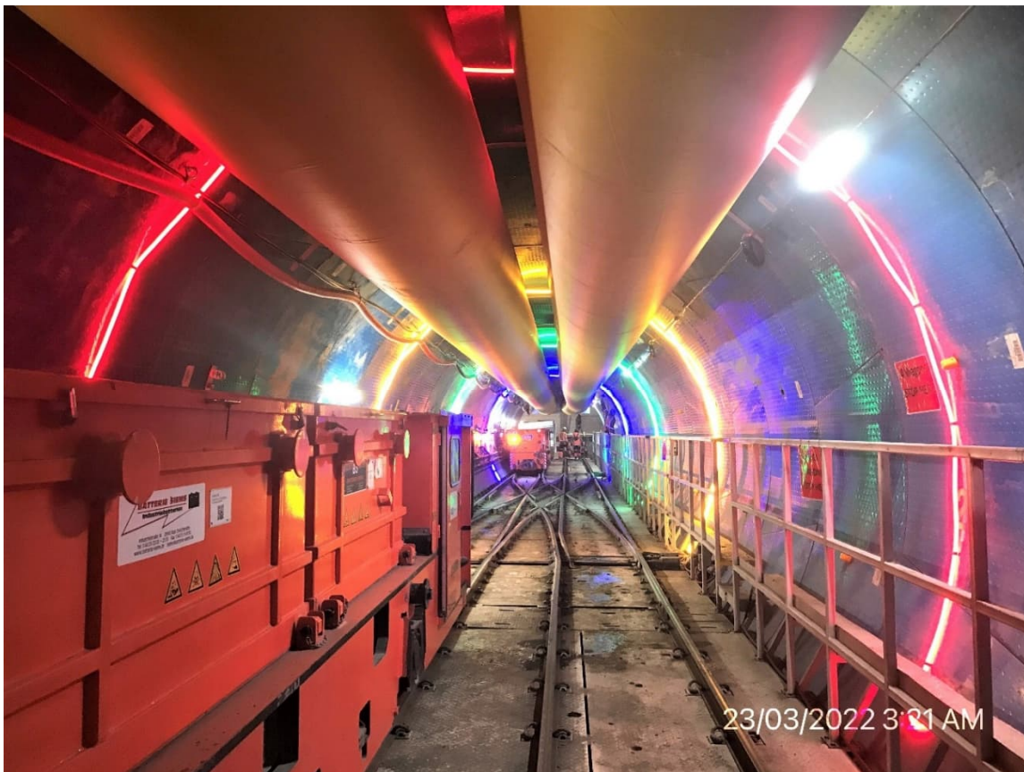
Figure 4.4: CI Tunnel March 2022 – tracks and bins for removal of spoil from the tunnel
