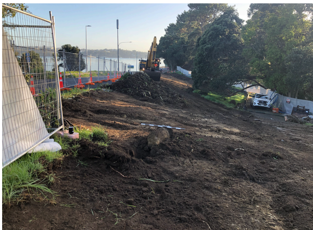
Figure 54. Topsoil stripping along the eastern face of the Curran Street on-ramp within Point Erin Park (June 2020)
