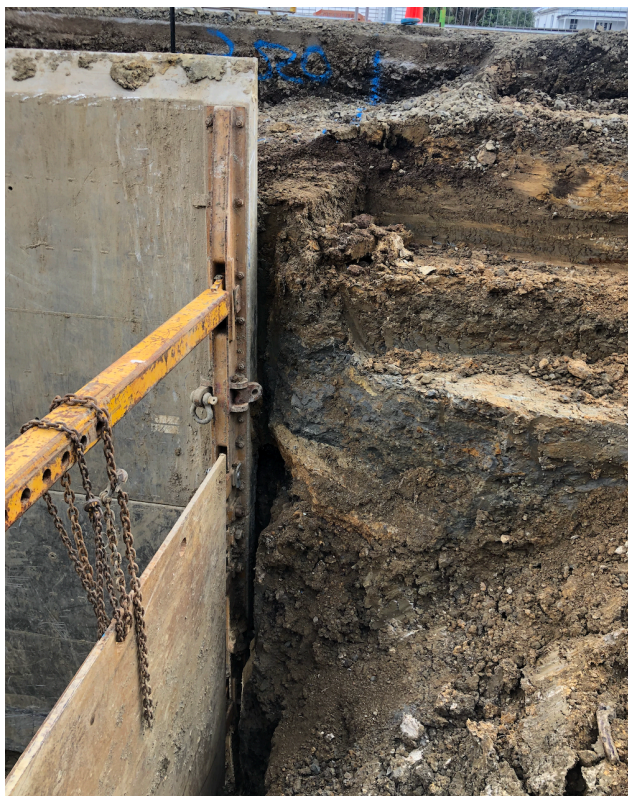
Figure 56. Side of 6m deep trench through mixed clay fill for the installation of a rising main and gravity pipeline (August 2020)
