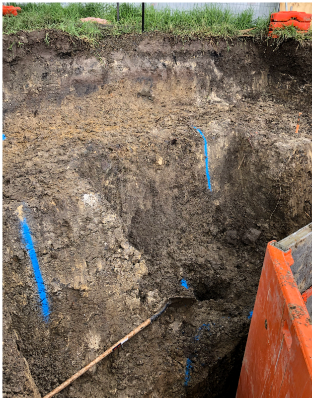
Figure 55. Excavation of the manhole chamber at the Point Erin Park pedestrian entrance through 5m of mixed clay fill (August 2020)
