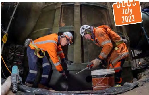
Installing shaft liners
