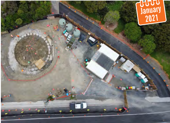
Secant piling: shaft
