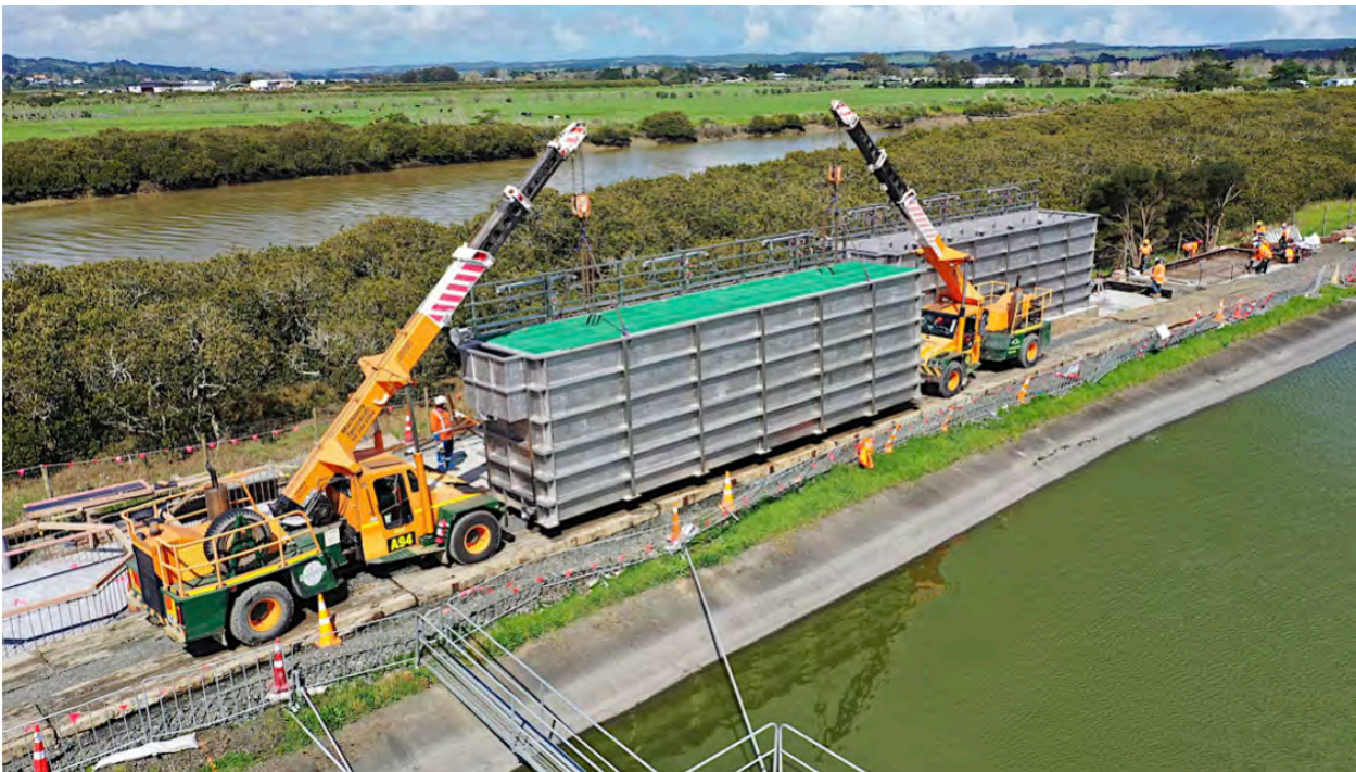
Figure 11 - Upgrading the Helensville Wastewater Treatment Plant
