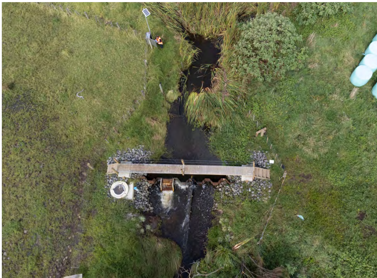
Helensville Water Treatment Plant 2023
