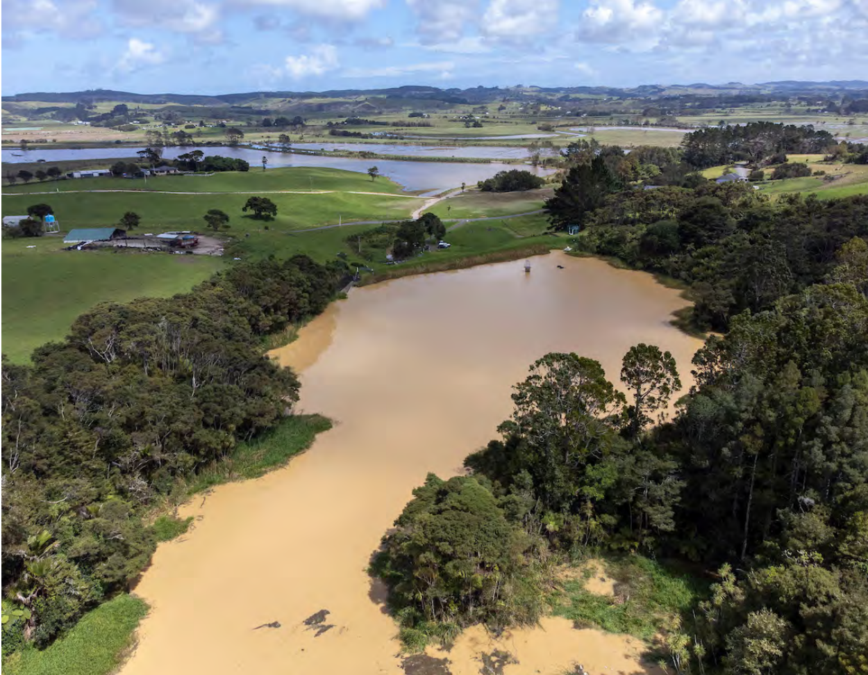
Helensville Dam Feb 2023
