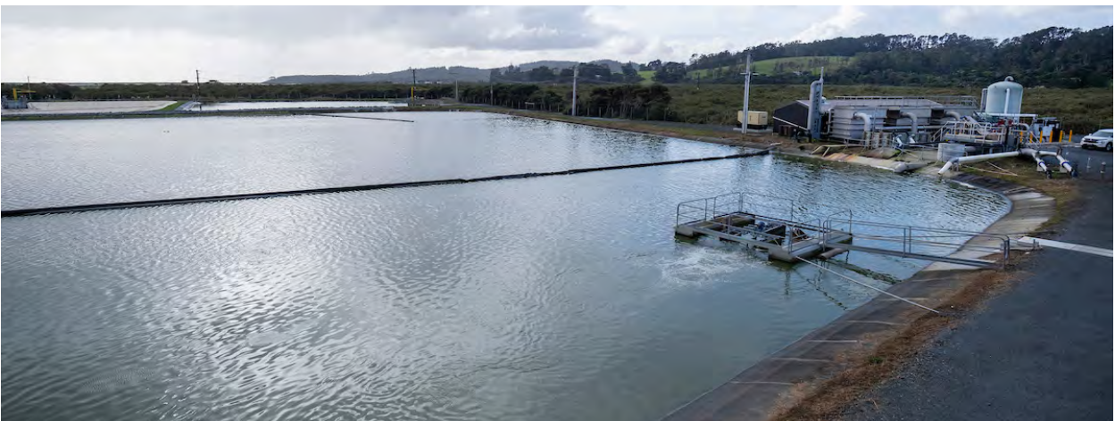
Helensville WWTP June 2023
