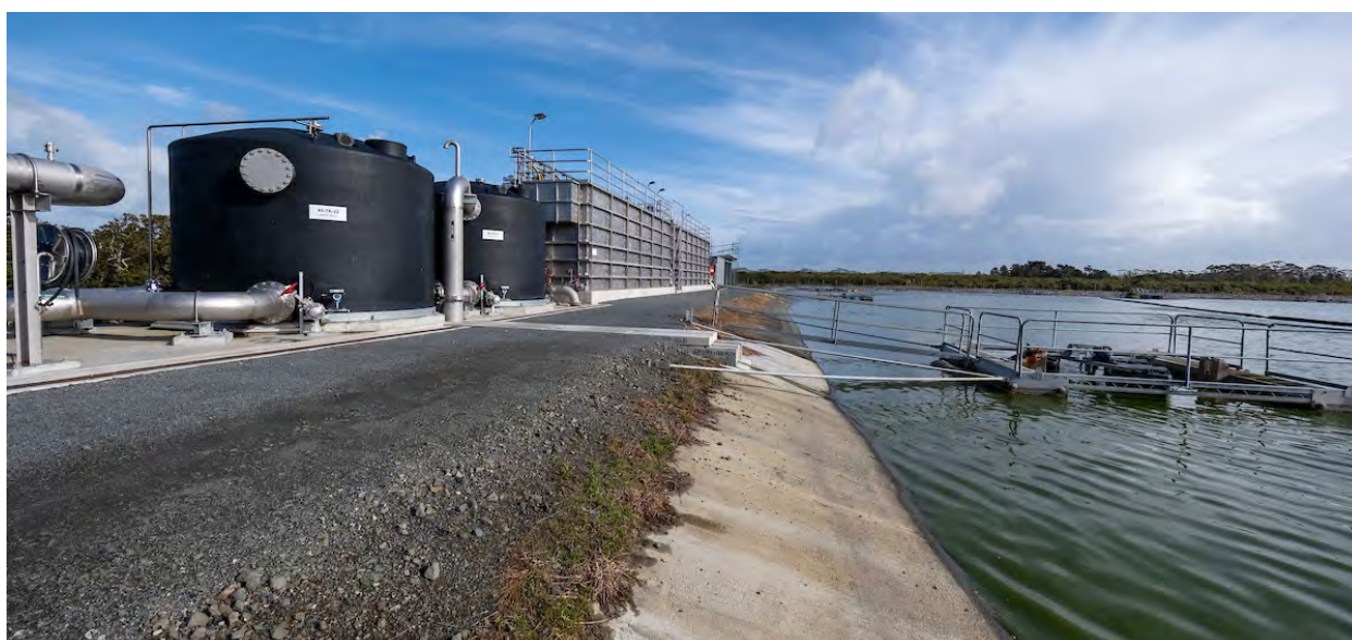
Helensville WWTP June 2023
