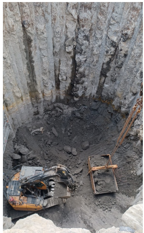
Figure 6 Typical Secant Pile shaft under Excavation
