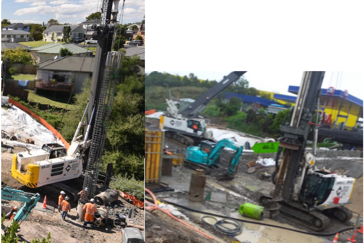
Figure 7 Typical Secant Pile construction
