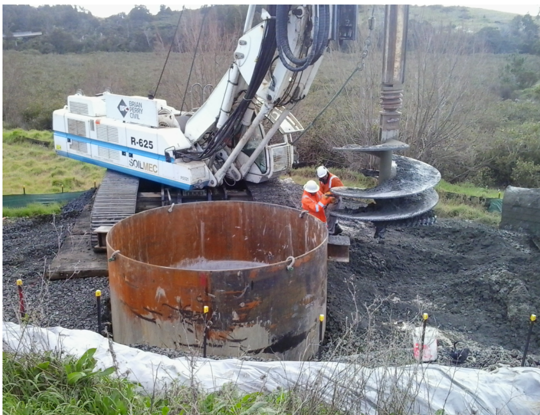
Figure 8 Interception shaft Casing installation
