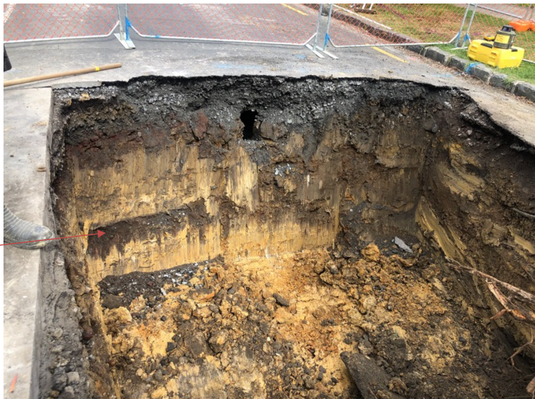
Figure 35. Trenching along the northern side of Sarsfield Street in 2020 adjacent to Point Erin Park. The buried old road surface of Sarsfield Streets is arrowed
