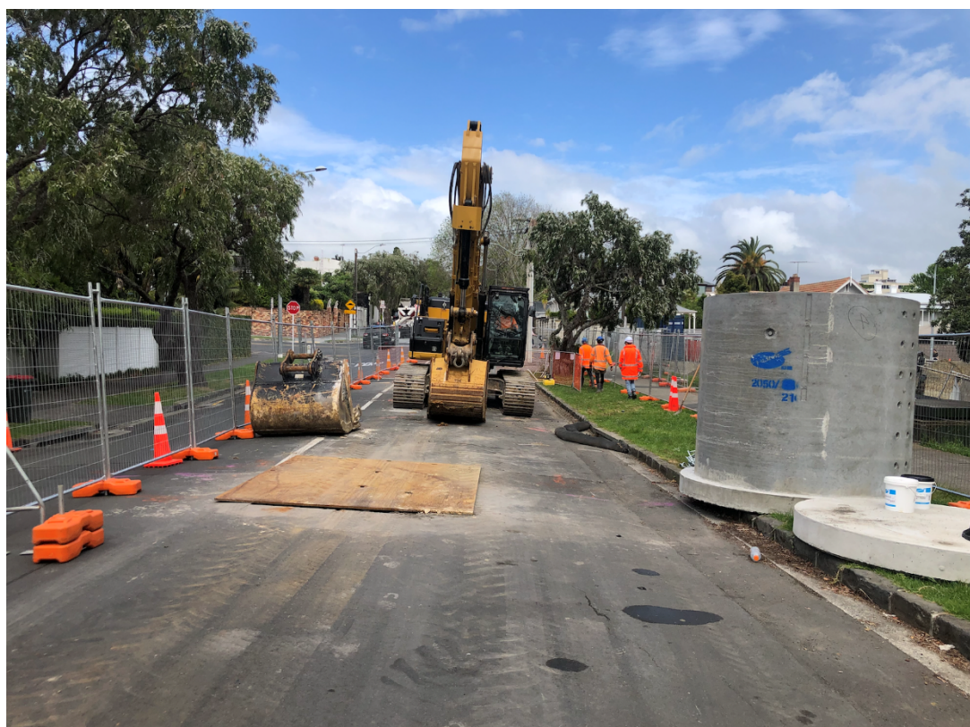
Figure 34. Trenching to install a gravity pipeline (Sarsfield overflow collector) along the northern side of Sarsfield Street in 2020 adjacent to Point Erin Park
