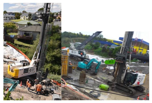
Figure 7 Typical Secant Pile construction
