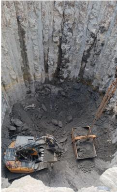
Figure 6 Typical Secant Pile shaft under Excavation
