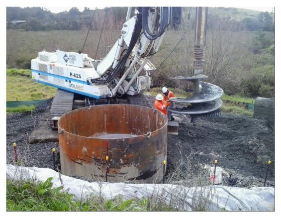
Figure 8 Interception shaft Casing installation
