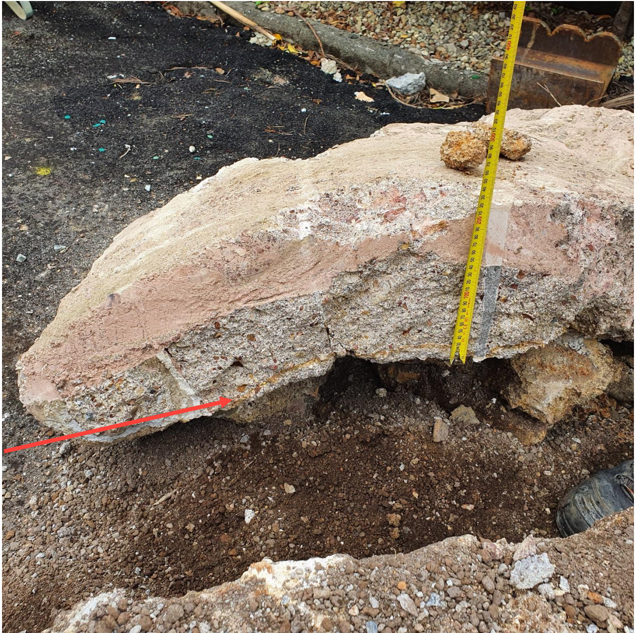
Figure 5 Typical block arch section after removal. Note the brown line indicating the extent of corrosion on the inside face (see red arrow).
