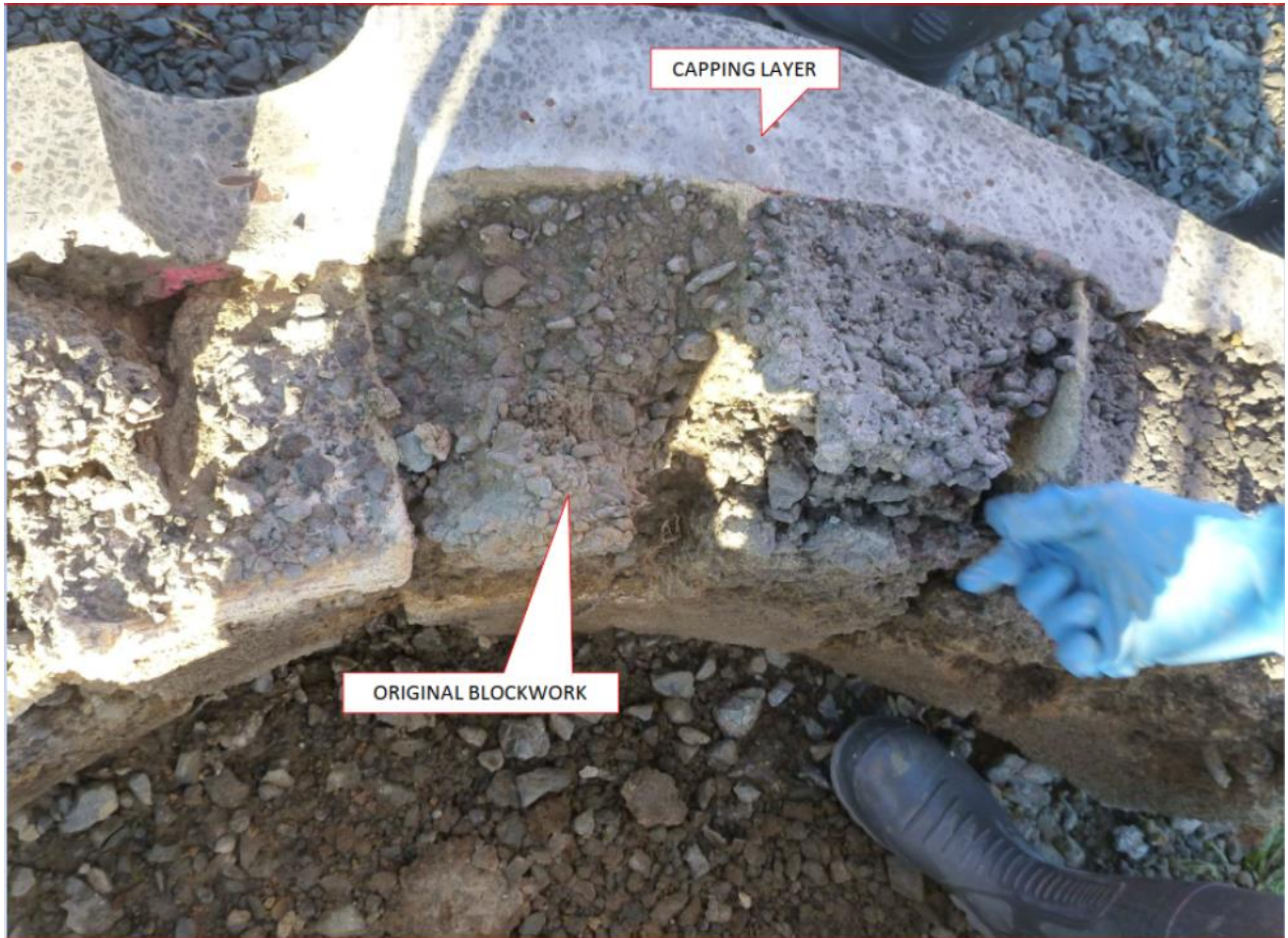
Figure 3:9 Photo of capping layer and original blockwork
