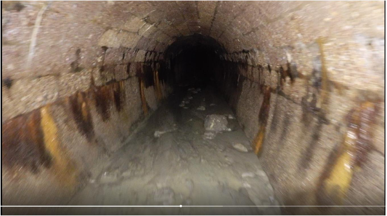
Figure 5 – General Condition of Sewer Between Manhole 15 & Manhole 14
