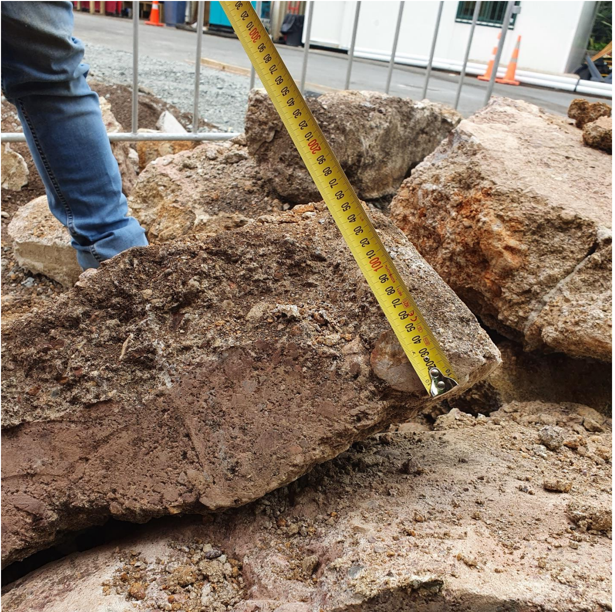
Figure 6 Measurement of concrete layer at edge of block arch
