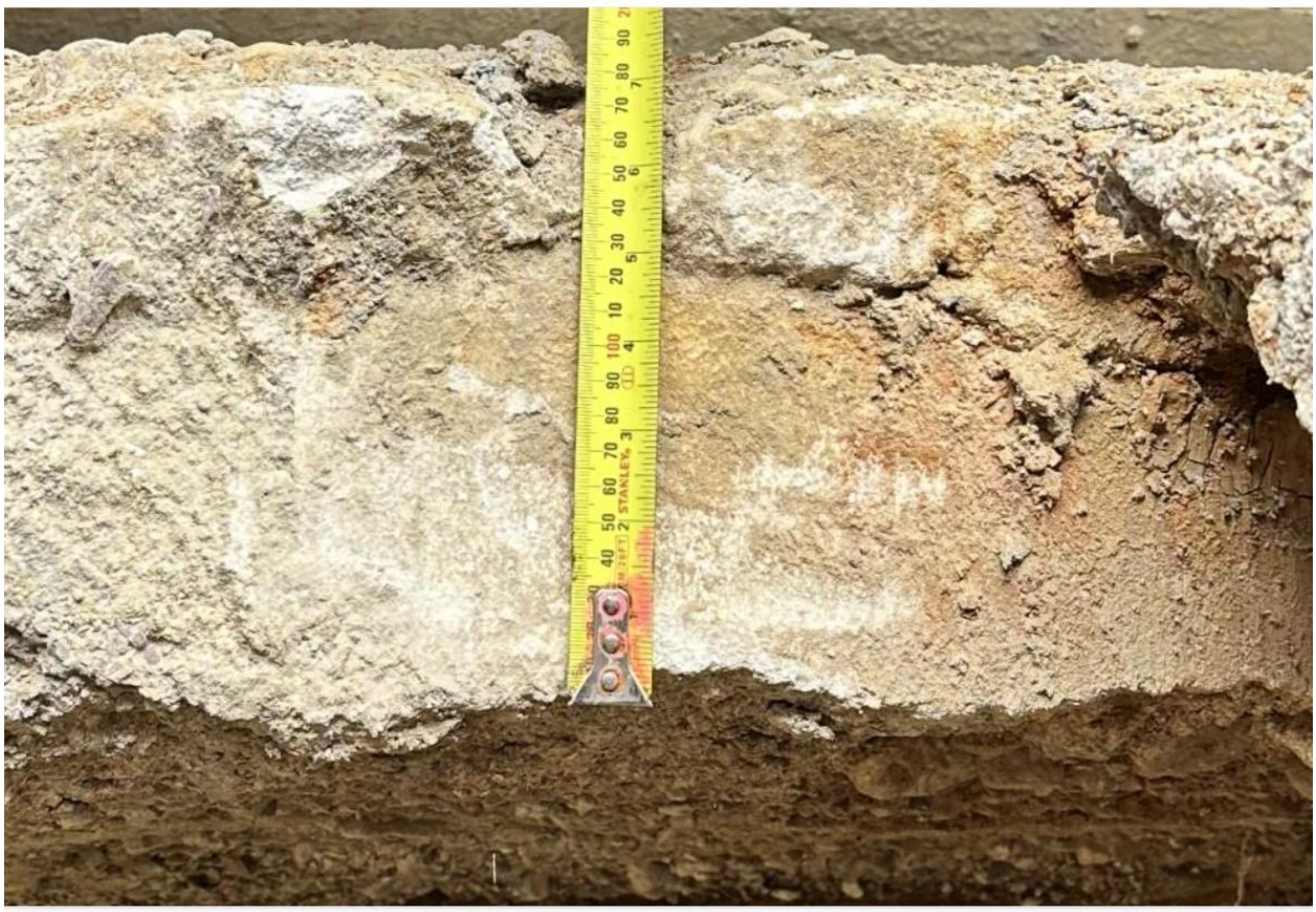
Figure 4 Typical block arch section in-situ
