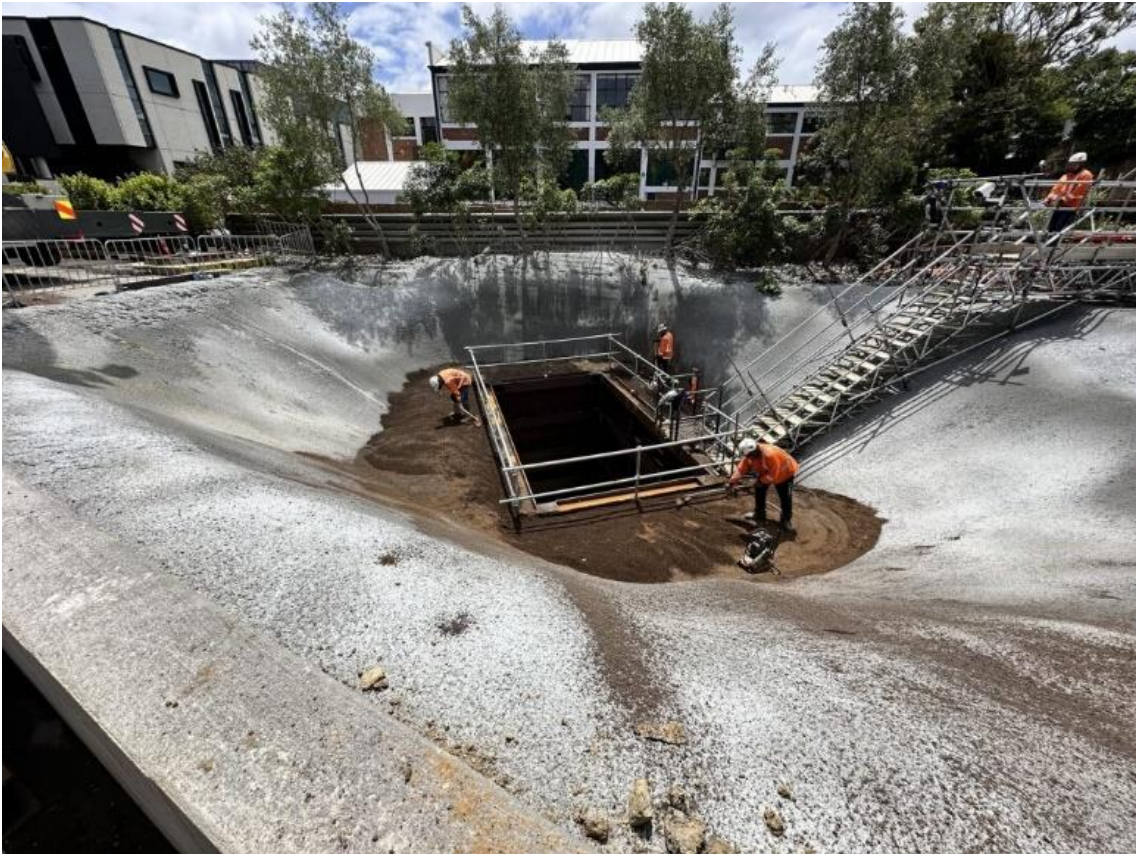
Figure 1 Trench Shield Installed over Collapsed Section of OMS
