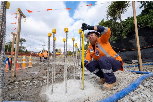
Dundale Ave – Site Engineer checking reinforcing bars for capping beam preparation
