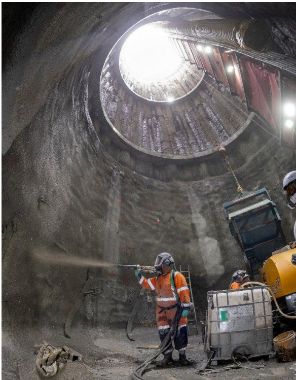
May Road – shotcrete being applied at the base of Shaft A
