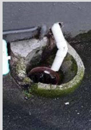
Broken gully dish allowing stormwater to enter the wastewater network
