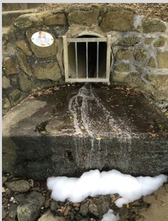
Soap, from window washing, discharging from a stormwater outfall onto Takapuna Beach.
