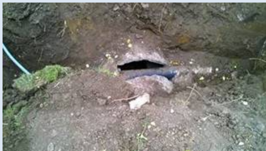
Takapuna toilet block - leaking wastewater pipe cutting through a stormwater manhole
