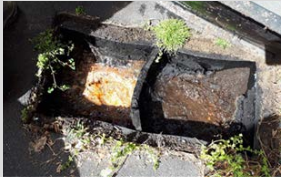
Private grease trap not cleaned
