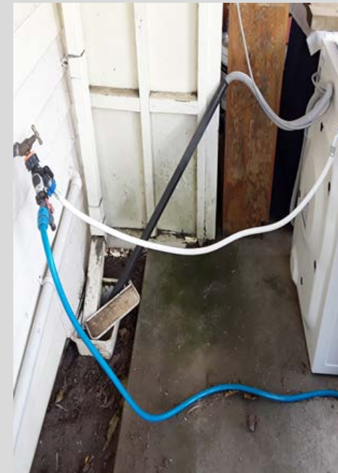
Washing machine illegally discharging into a stormwater pipe
