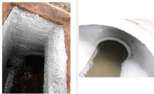
Wastewater pipe cleared of tree roots and relined
