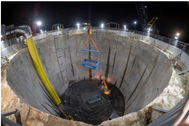
MPS – Main Shaft excavation
