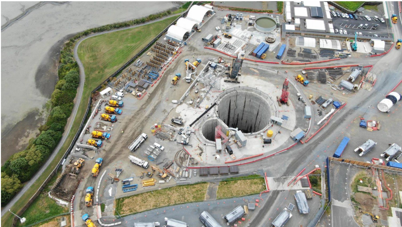
MPS - Main shaft base slab concrete pour in progress
