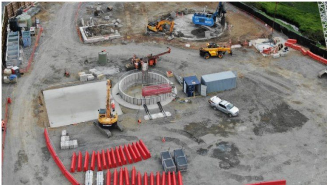
May Road - Shaft A preparation for excavation/mine site setup
