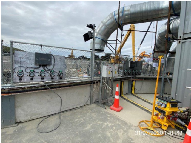
MPS – Ventilation and air quality monitoring ready for shaft excavation
