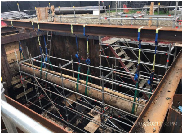
Keith Hay Park – Support of Branch 9A sewer for construction of diversion chamber
