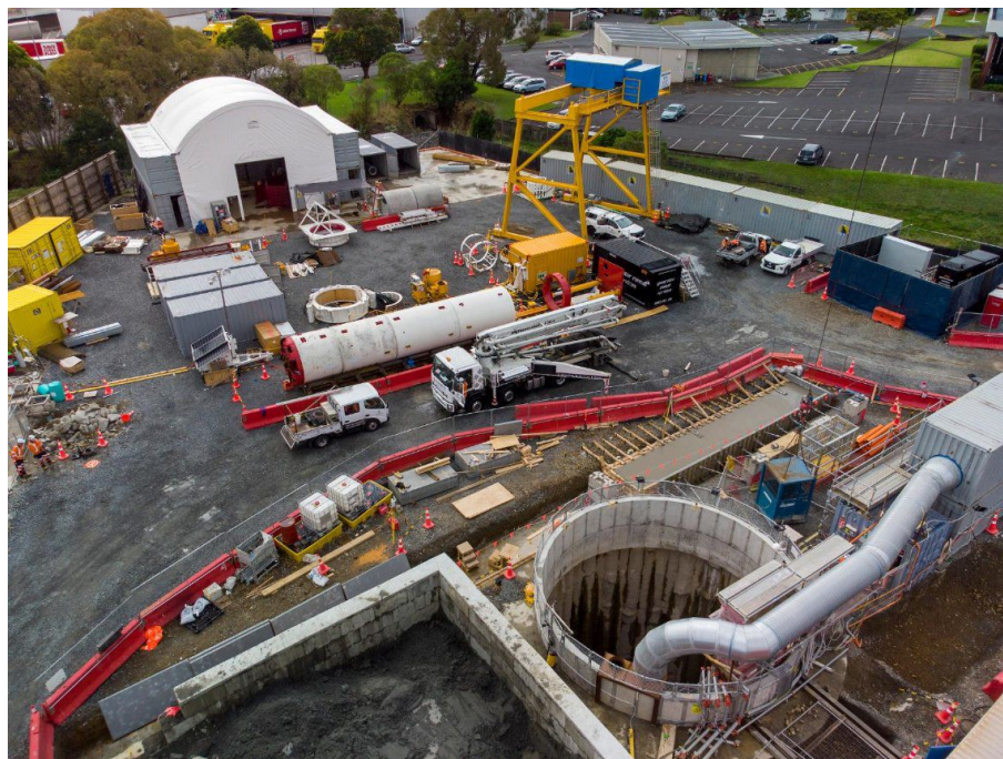
May Road – Shaft A and MTBM assembly
