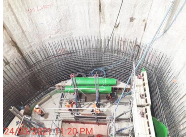
MPS – Inlet shaft, installation of reinforcing steel for permanent wall construction
