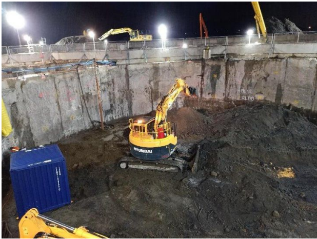
MPS– Main Shaft excavation
