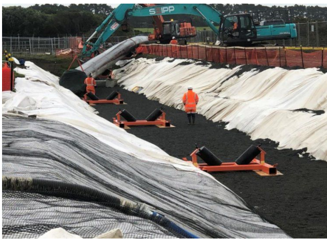
MPS – Laying rising main pipe in trench
