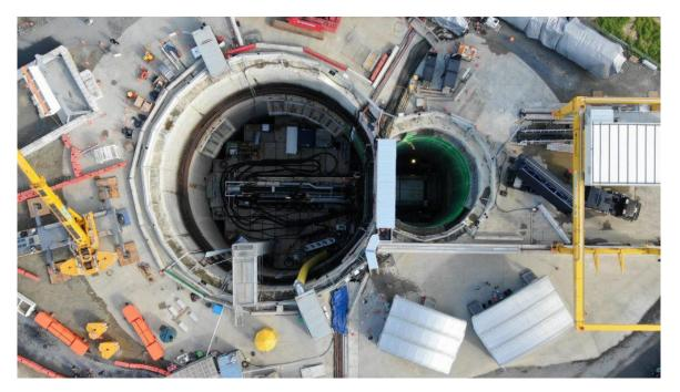
MPS – TBM (including gantries 1 & 2) assembled at the base of the shafts
