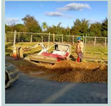
A 1.7 tonne excavator was inside a trench, being used to spread metal during a backfilling operation. As the excavator was reversed out of the trench, the operator tracked over the metal ramp that was uneven and not properly compacted. This caused the right track of the digger to sink into the metal, tipping the excavator 70 degrees onto its side, resting on the edge of the trench.
