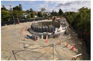
May Road – Drilling in preparation for rock bolt installation
