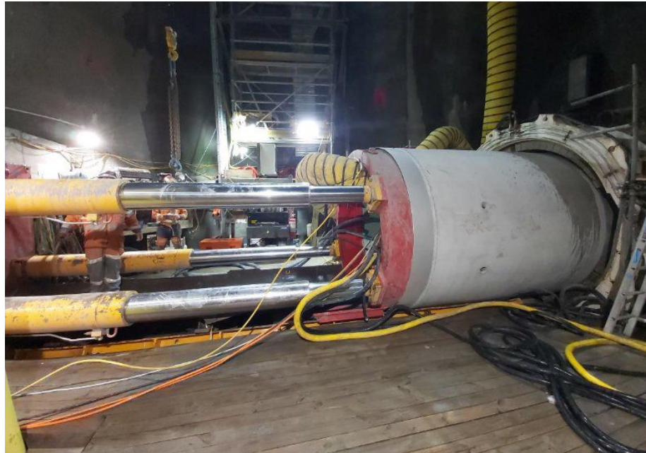
May Road – Hydraulic rams pushing jacking pipe for Link Sewer C drive to Haycock Ave
