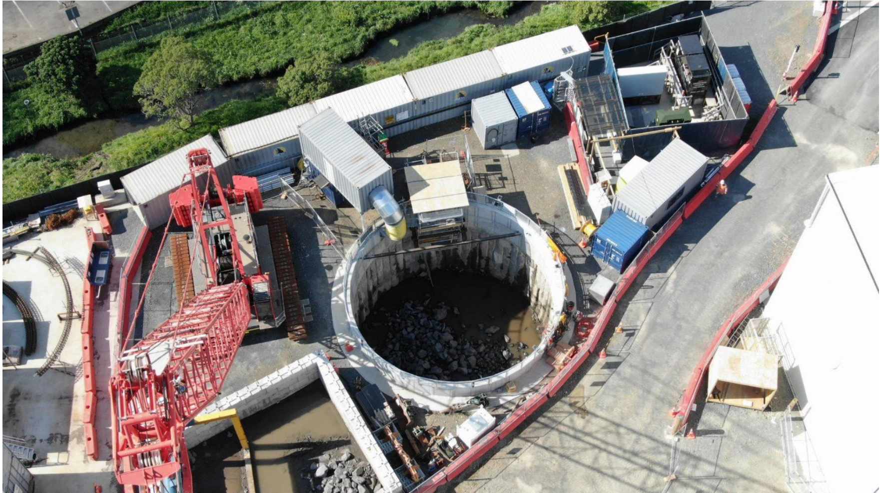
May Road – Shaft B excavation
