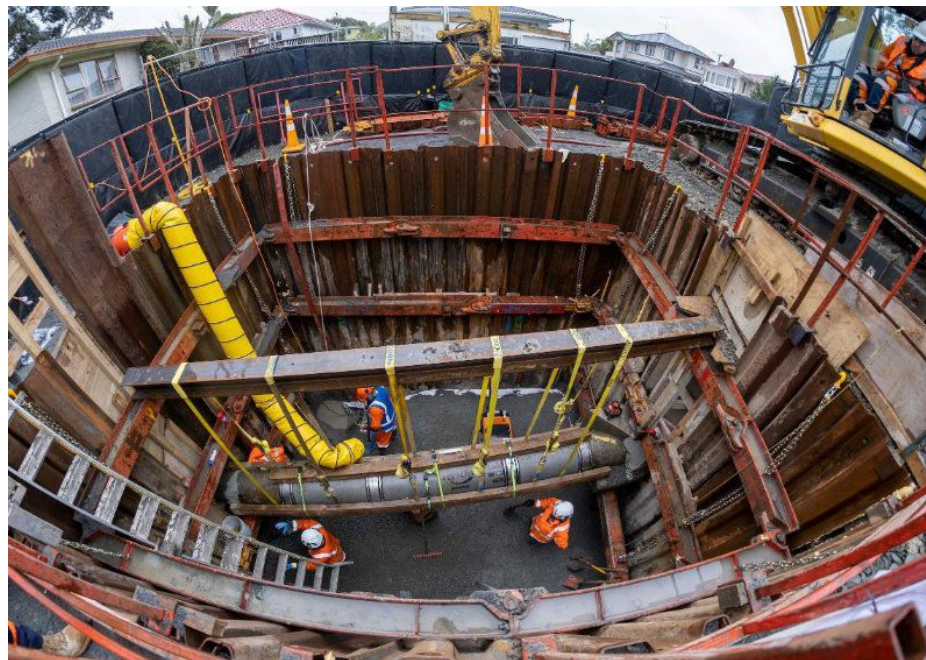
Haycock – Replaced section of Lynfield Branch Sewer
