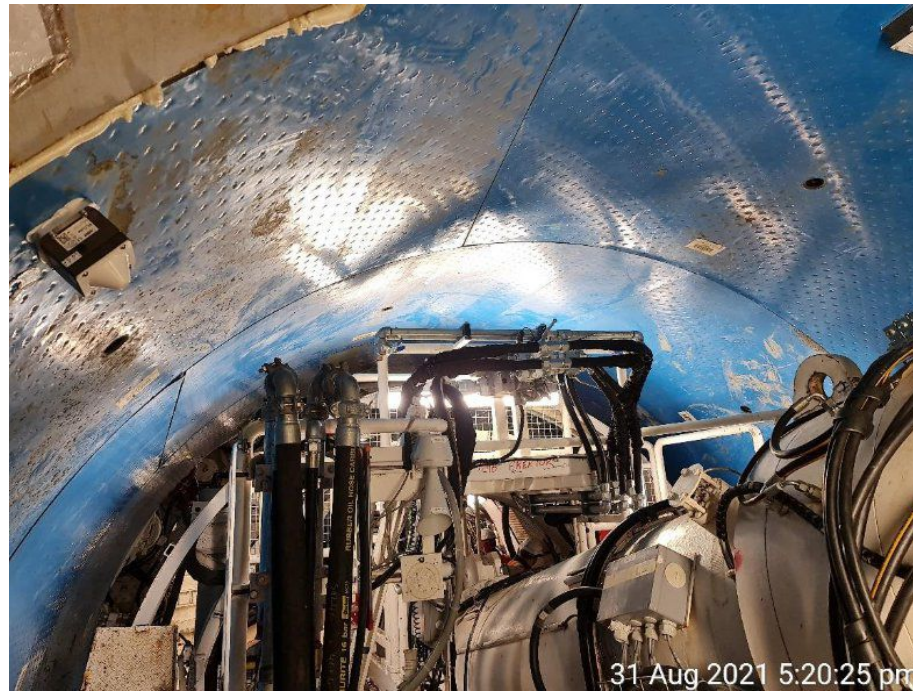
Main Tunnel – First three rings installed
