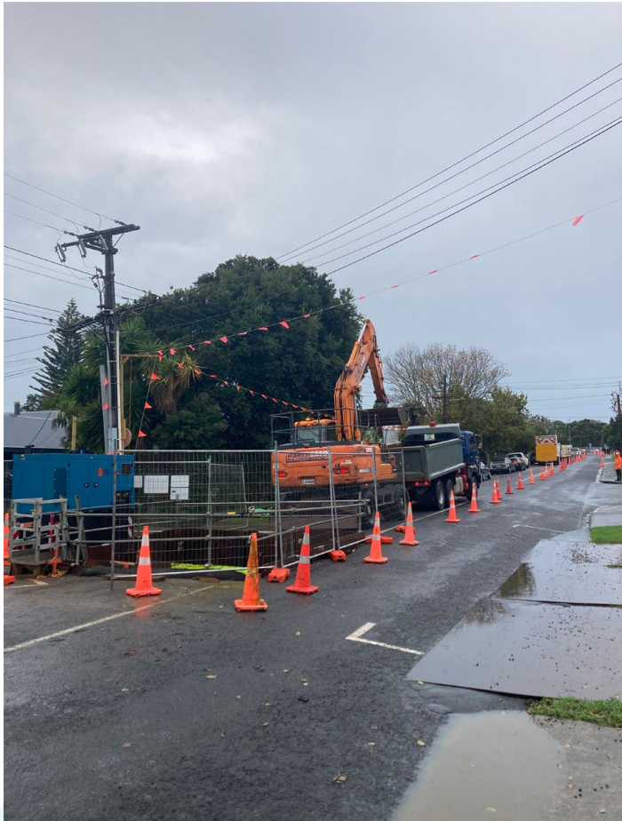
TARP PS Rehab Yr1 – Alma Road – exclusion zones, overhead power line flags
