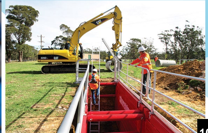
Trenching – edge protection and safe access
