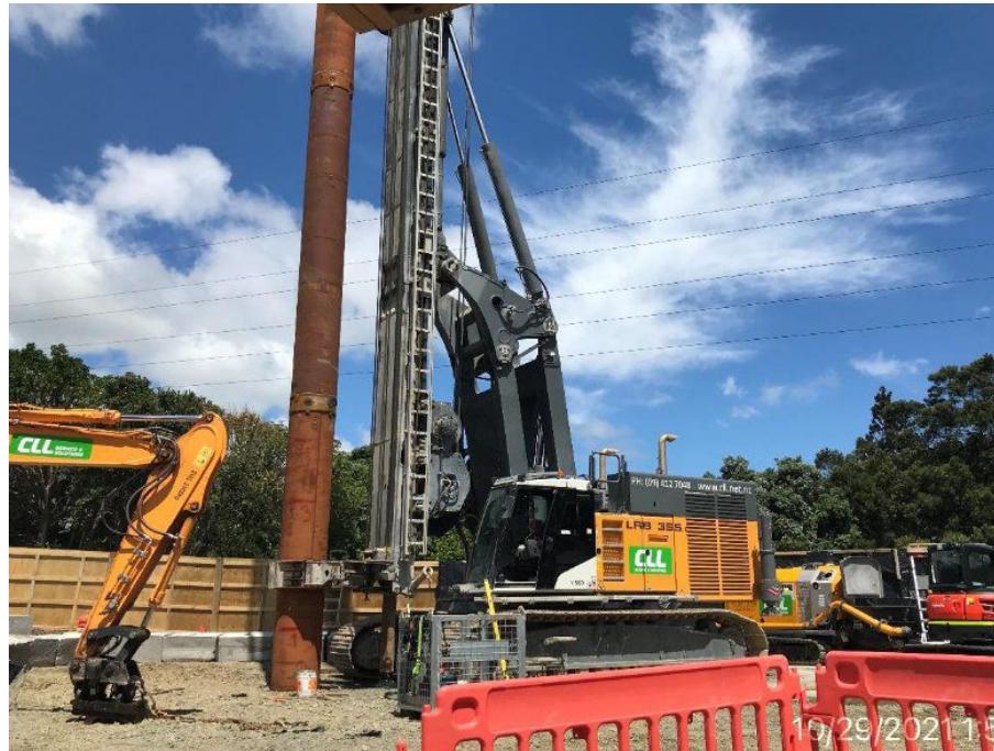
Miranda Reserve – piling rig on site to install secant piles
