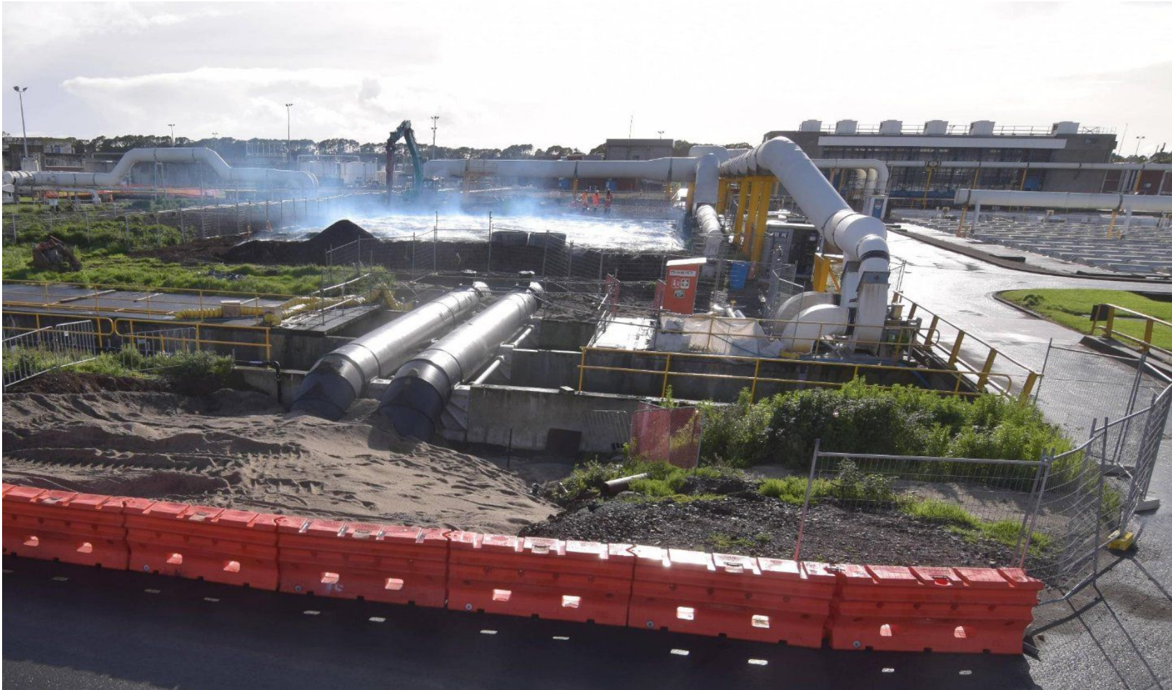
Māngere Pump Station – rising main / Odour Bed 4 Smoke Test
