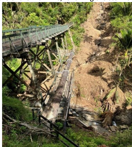
Slip adjacent to Quinns Bridge – damage to pipebridge, Tramline bridge to be inspected
