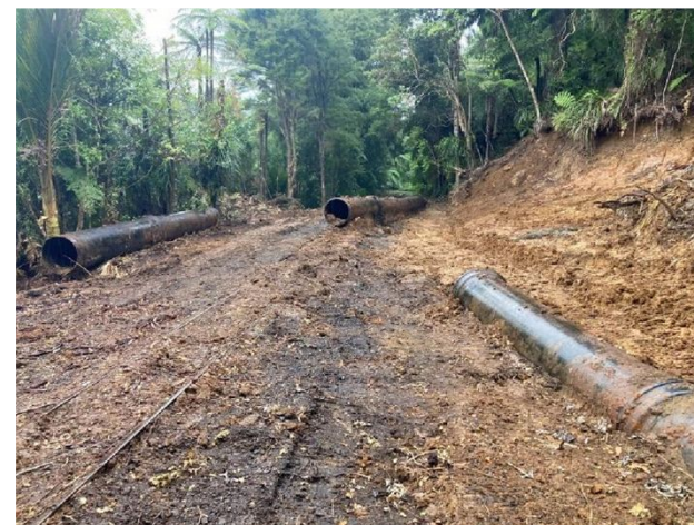
Upper Nihotupu Raw Water Main displaced by slip which covered Tramline, repair underway
