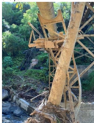
Slip adjacent to Quinns Bridge – damage to pipebridge, Tramline bridge to be inspected
