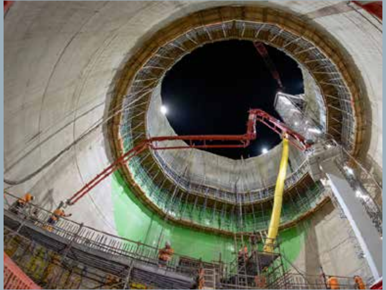
Pouring concrete inside the Māngere main shaft
