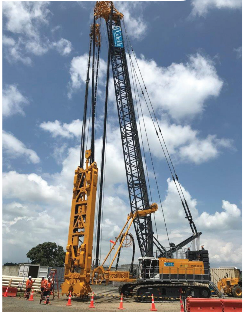
The hydrofraise cutterhead being readied for operation
