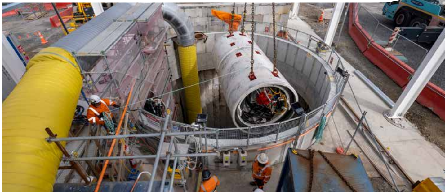
The mTBM being lowered into Shaft A.
