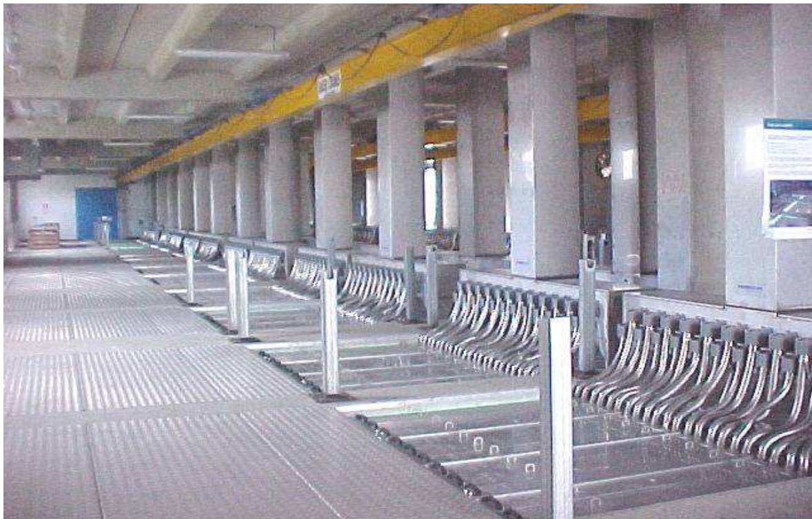
Figure 6 The Mangere WWTP UV Disinfection System
