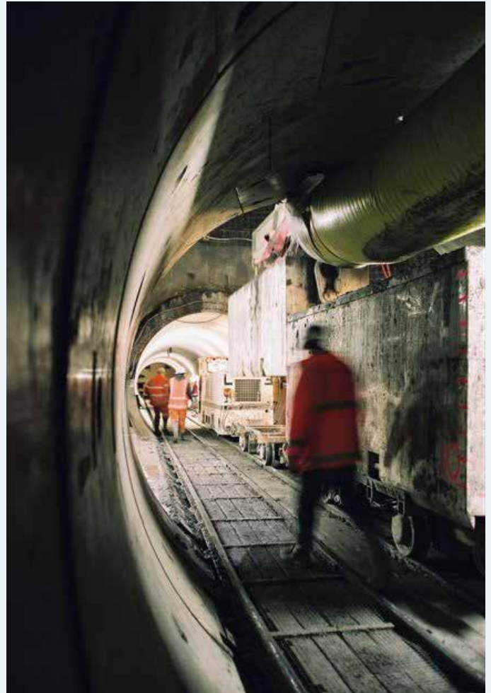
Hobson Bay tunnel construction.
