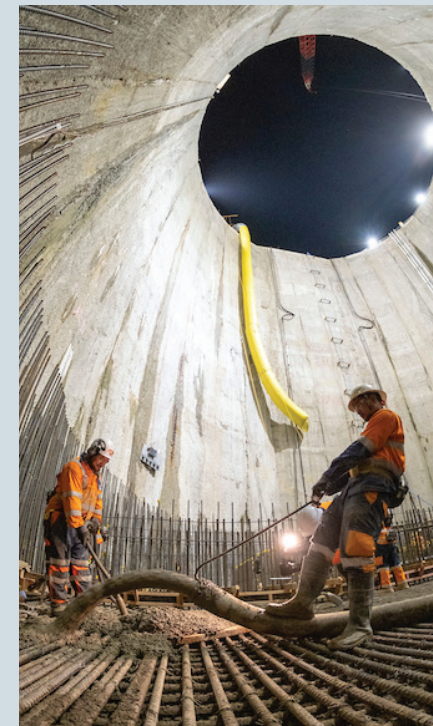
Late night concrete pour 42m down in the Māngere main shaft just before Christmas.
