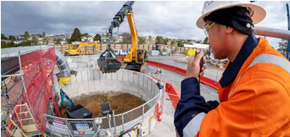
John 'Jeck' Mallari, high in position at May Road. Jeck is shown working as a dogman on the safe rigging of the load and directing of the lifting and placing operations of one of our excavators. Jeck is a leading hand on site and will soon complete his B grade Tunnel Managers Certificate.
