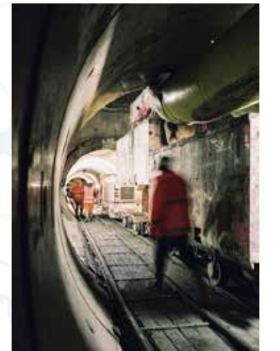
Hobson Bay tunnel construction.
