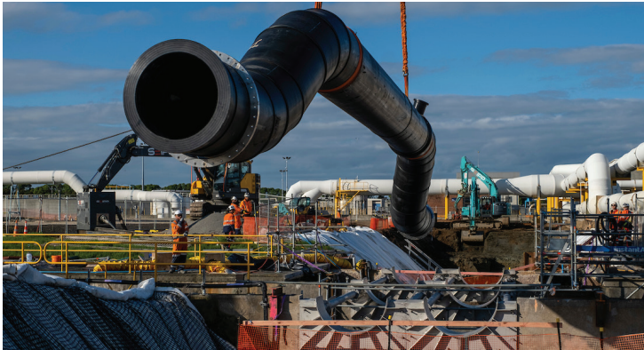
A section of the 1.6m-diameter polyethylene rising main being lifted into place
