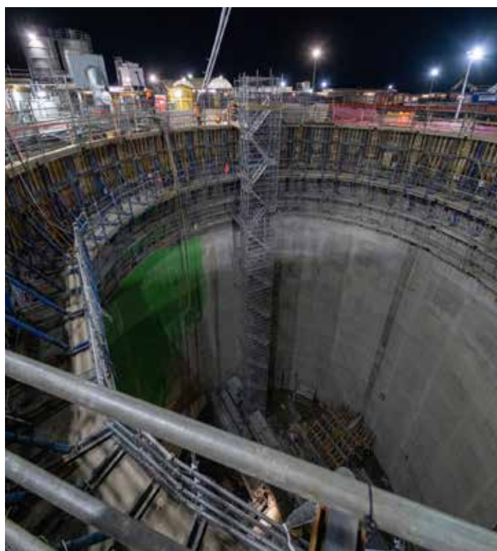
Lining the pump station shaft with concrete
