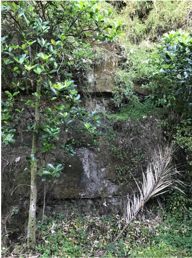
Figure 3.3: Thickly and horizontally bedded volcaniclastic sandstone seen on the inside of the Exhibition Drive cutting immediately upslope of Reservoir No. 1.
