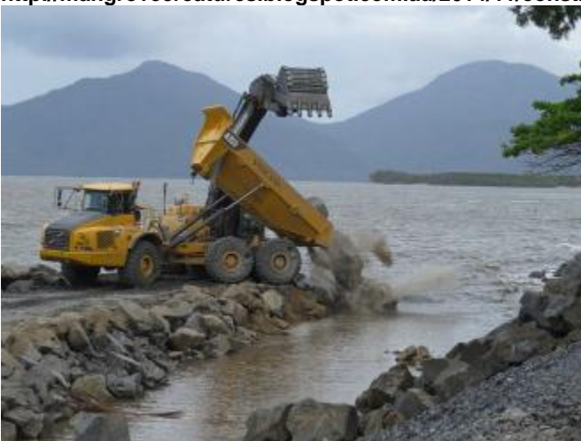
Figure 2-13: End-tipping used on the Machans Beach Seawall (source: http://mangrovecreatures.blogspot.com.au/2014/11/constructing-machans-beach-seawall.html )
