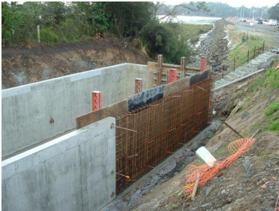
Figure 2-18: Assembly of pre-cast concrete walls (example from existing stormwater chamber adjacent to the causeway)
