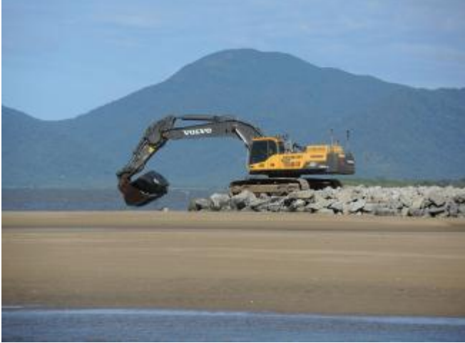
Figure 2-14: End-tipping used on the Machans Beach Seawall (source:
