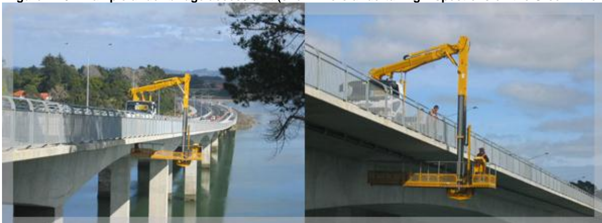
Figure 2-15: Example under-bridge access unit (shown here undertaking inspections on the Greenhithe Bridge)
