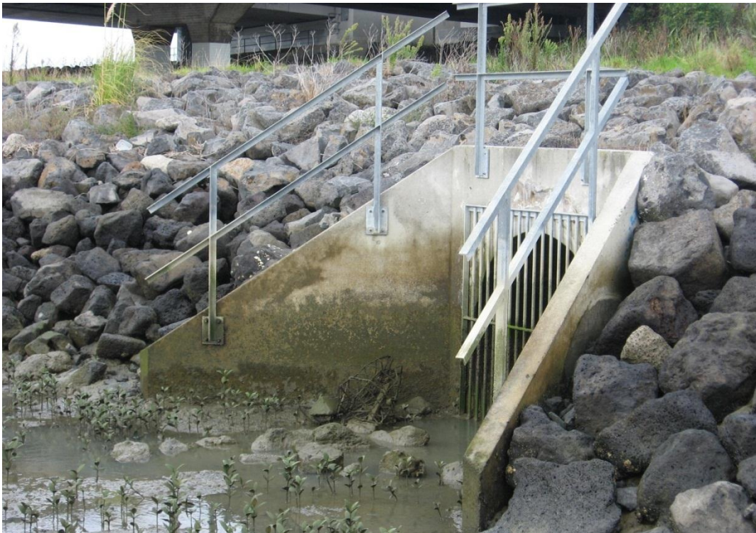
Figure 2-3: Example of outfall and rip-rap erosion protection below the Mangere Bridge
