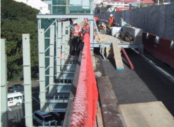
Figure 2-16: Example of movable scaffolding used on a similar project (the Khyber Pass Viaduct)
