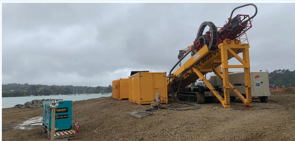
Site set up for the start of the horizontal directional drilling (HDD) at the Causeway.
