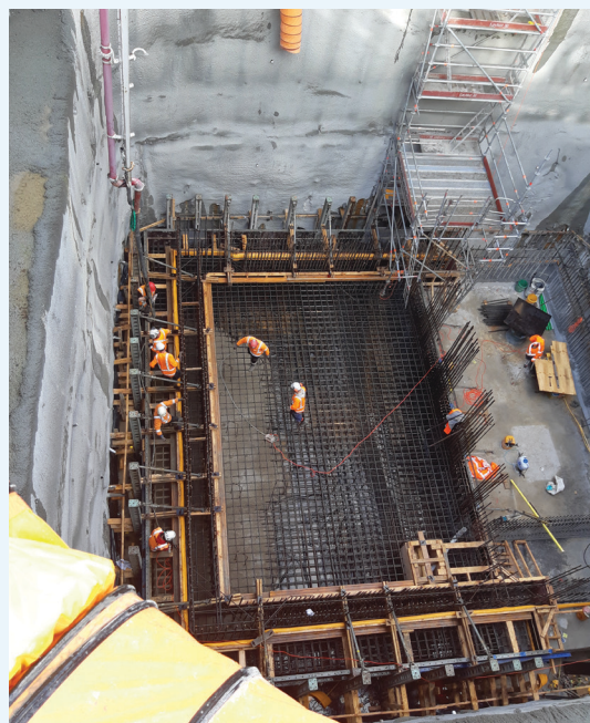
The concrete floor of the pump station being laid.
