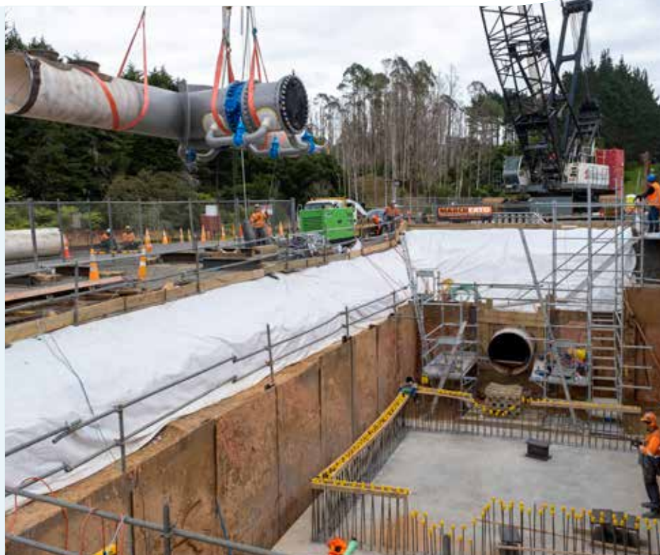
Preparatory work on the Waikato watermain was carried out in late-December 2020 to increase the volume of water that can flow through the pipeline to 225 million litres a day.
