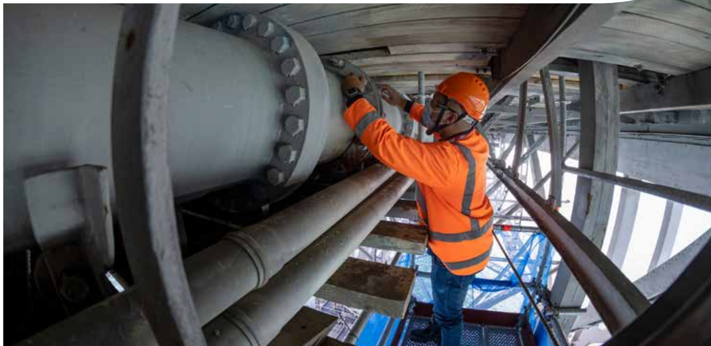
Watercare network engineer Alex Talakai Puloka realigns the joints on one of the pipes tucked under the Auckland Harbour Bridge to stop it from leaking.
