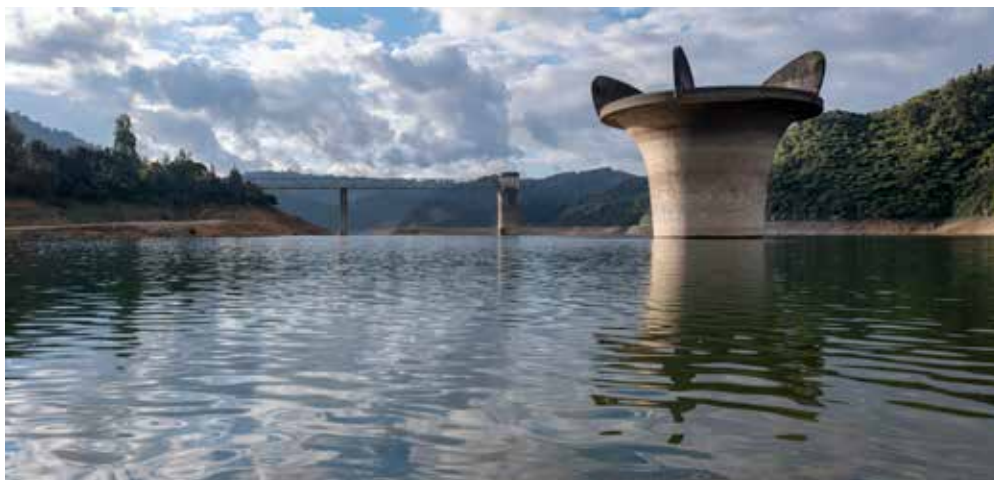
The spillway and valve tower are visible at Mangatangi Dam in the Hūnua Ranges.
