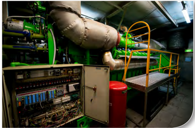
Methane gas generates engines to produce two-thirds of the energy at Mangere Wastewater Treatment Plant.
